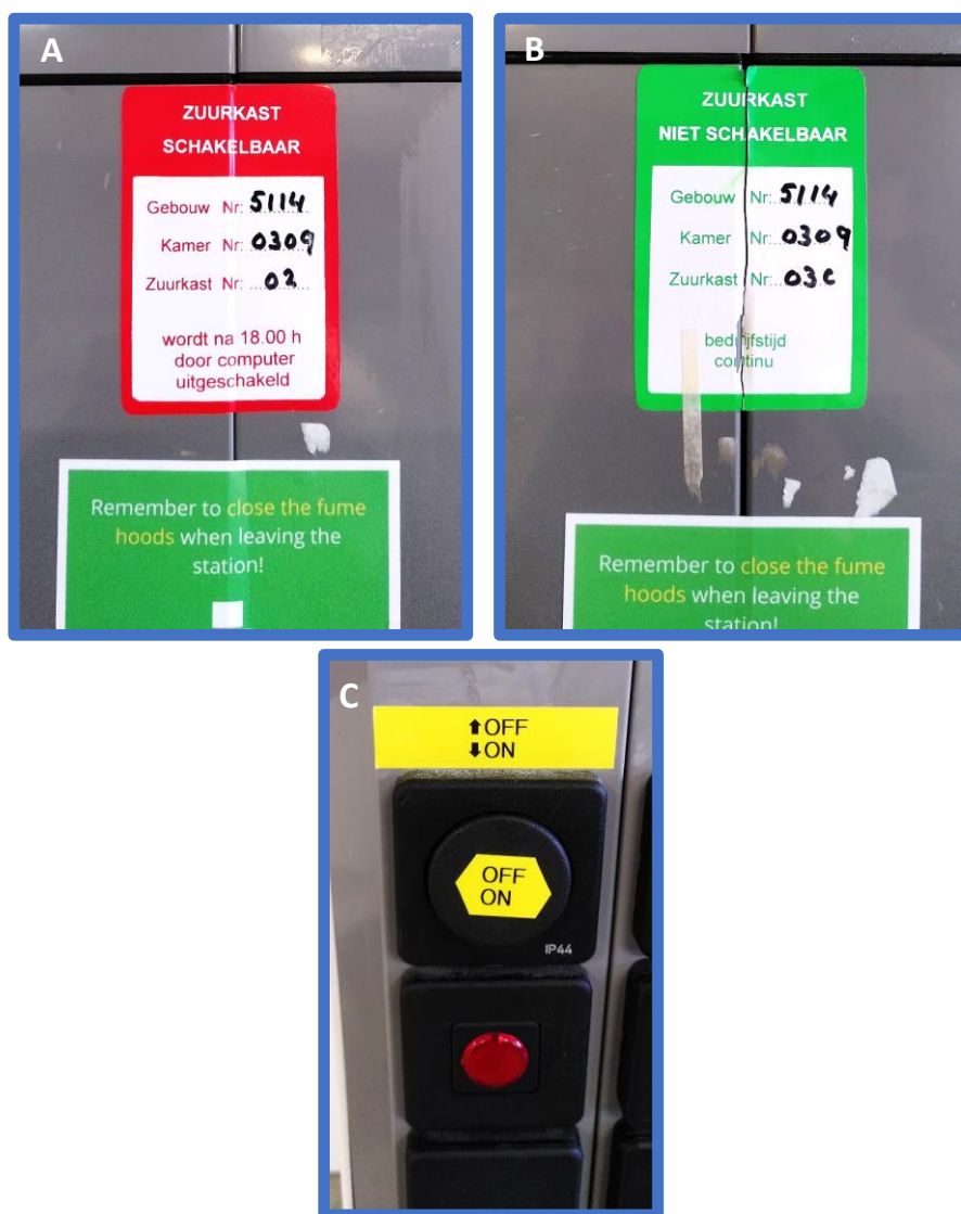
Figure 16: a) Some fume hoods automatically reduce airflow overnight. b) Sometimes due to air pressure and heating requirements of the building some fume hoods need to stay on during the night. c) Depending on the manufacturer there is also the possibility to manually turn off the fume hoods.
